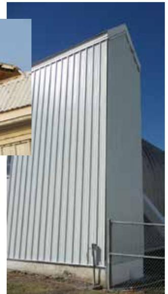
*Top left: This narrow image shows the deterioration of the existing metal siding on the north hangar doors bay.*
